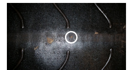
Failed Belt Wrap - Worn.
