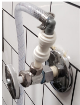
Figure 2. Output Water Valve with 3/8" OD Beverage Tubing
